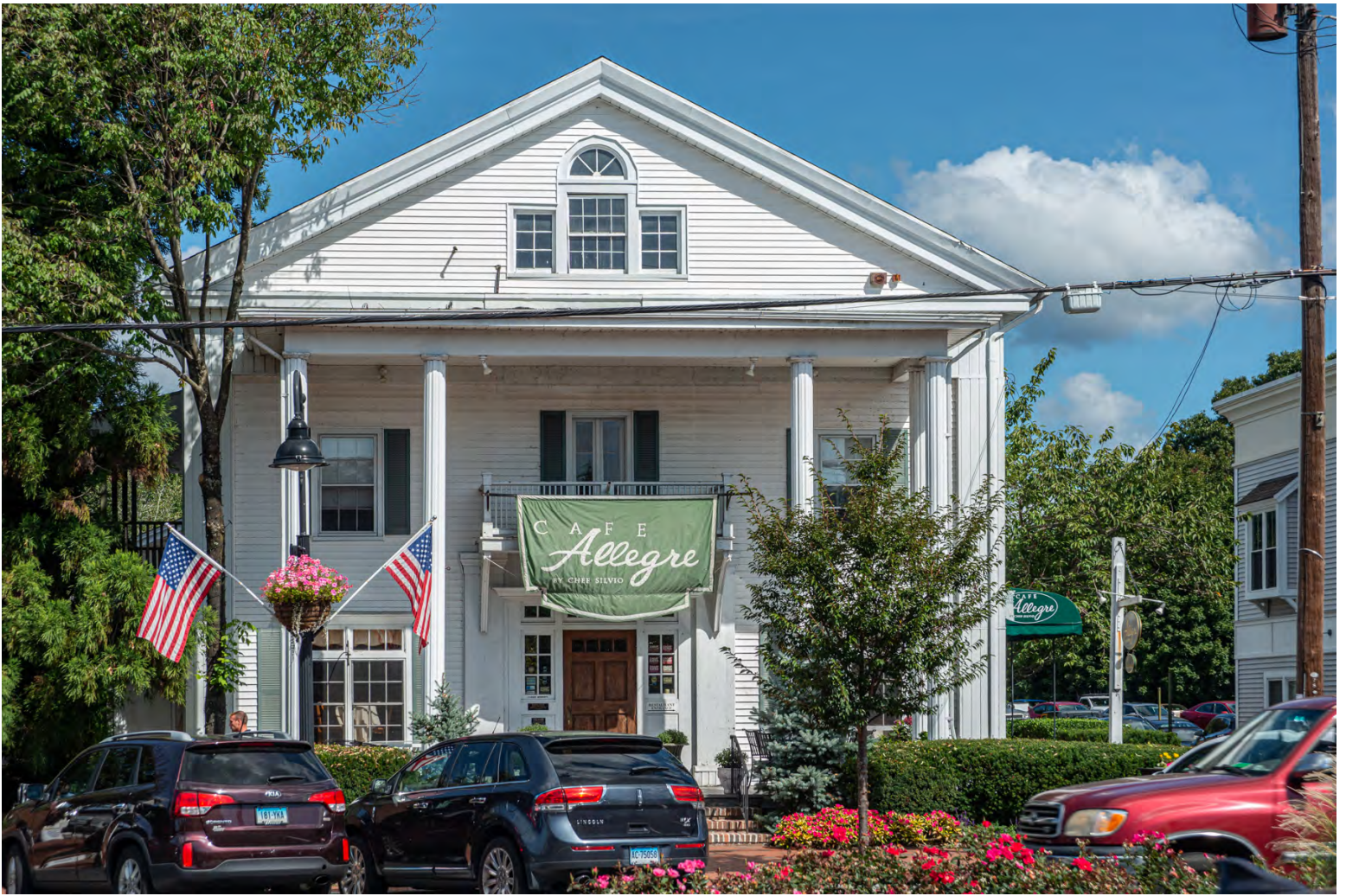
Photo 1. View north showing facade.
