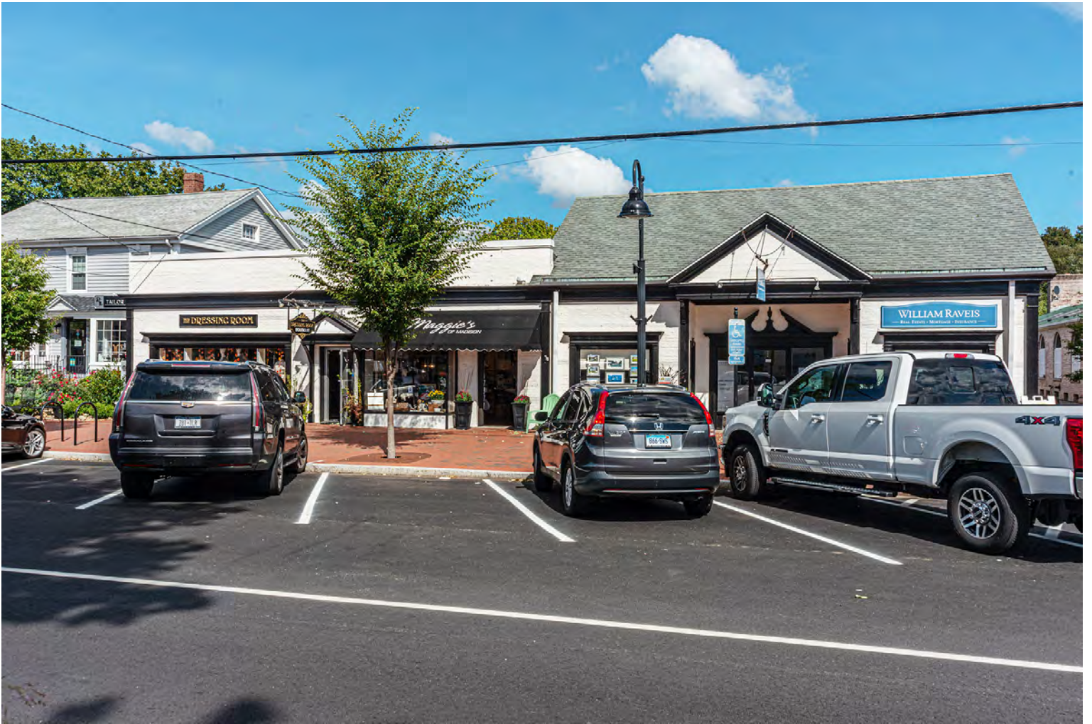
Photo 1. View north showing facade.
