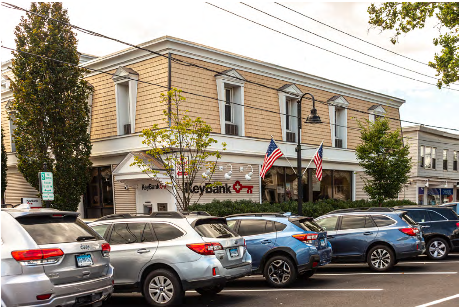
Photo 1. View southwest showing part of east elevation and facade.
