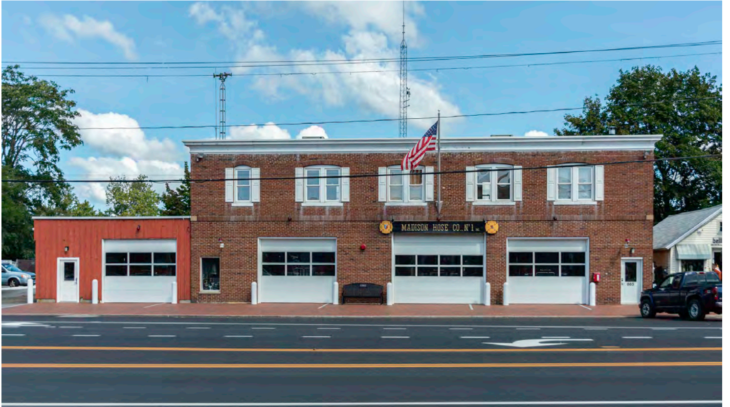
Photo 1. View north showing facade.
