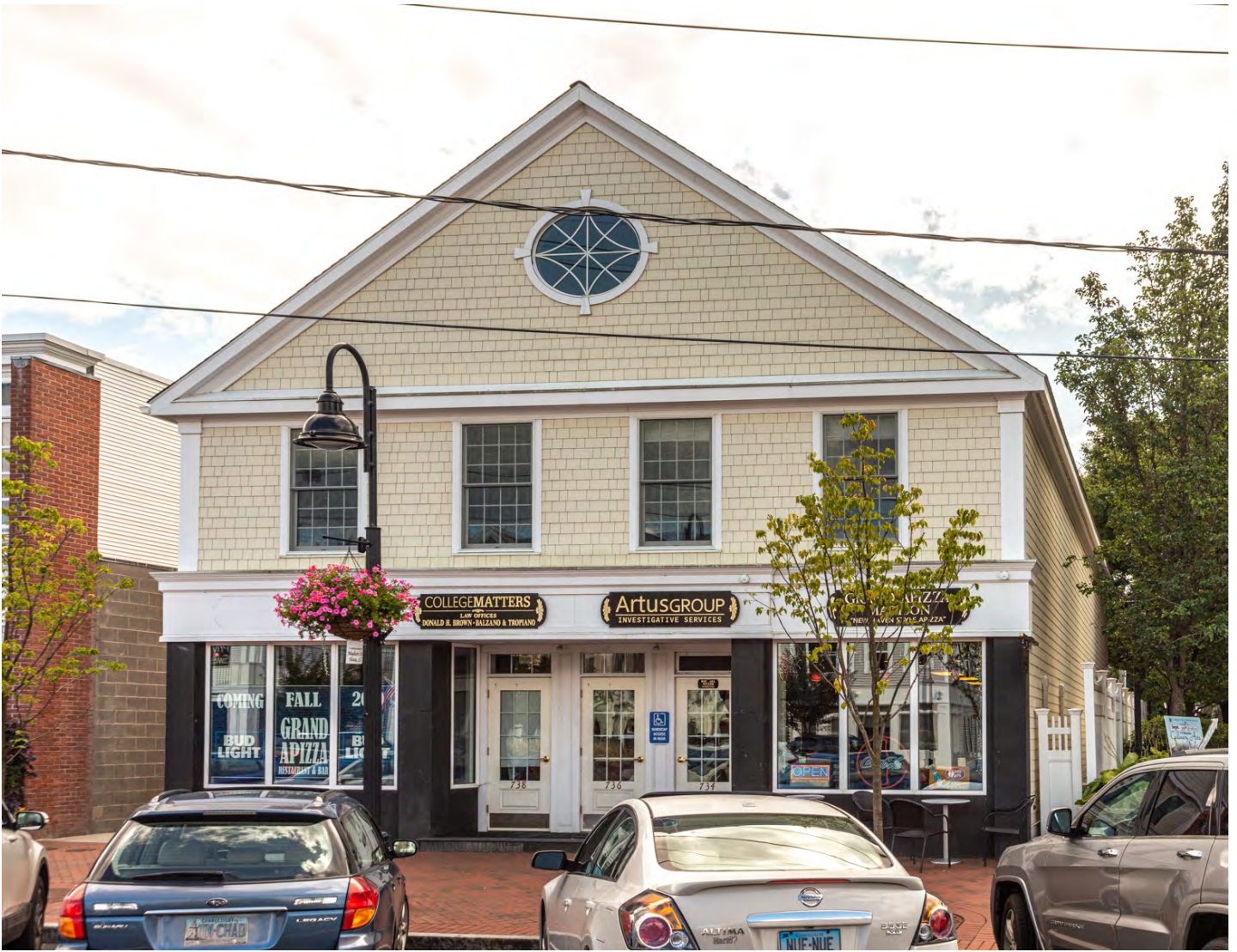
Photo 1. View South showing facade and part of west elevation.
