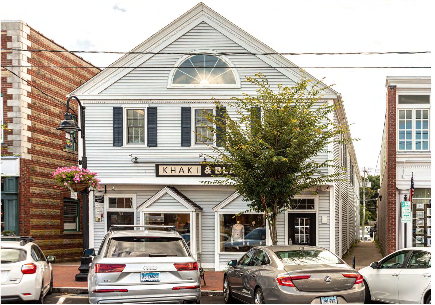
Photo 1. View south showing facade.
