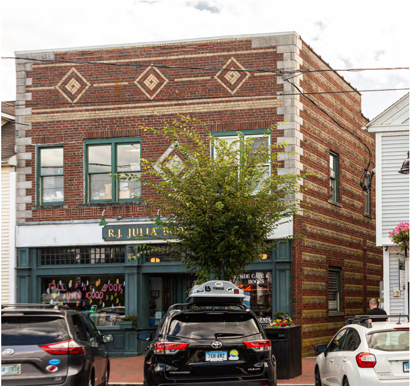
Photo 1. View southeast showing facade and west elevation.
