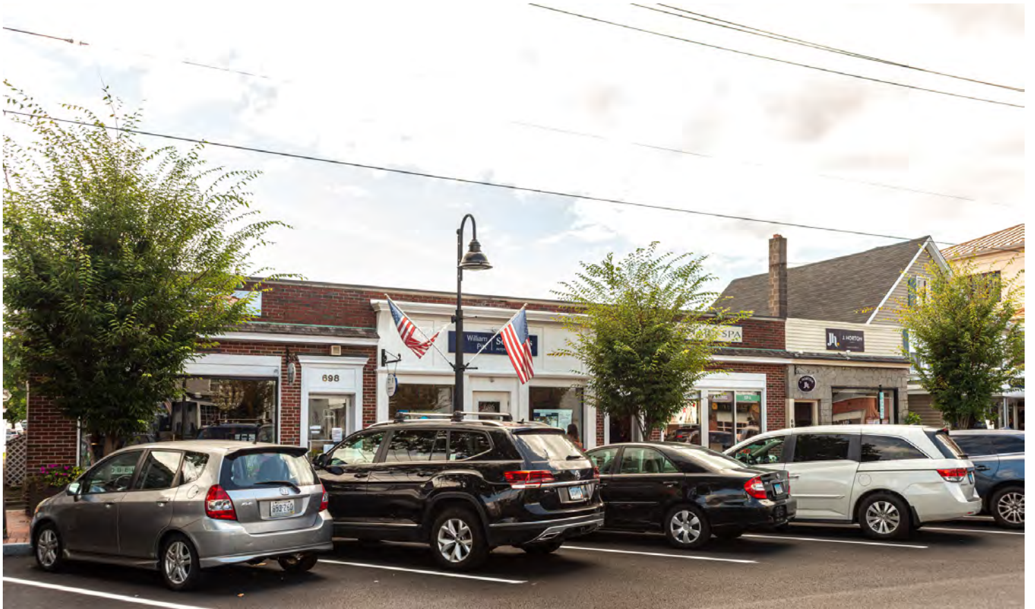
Photo 1. View southwest showing facade.
