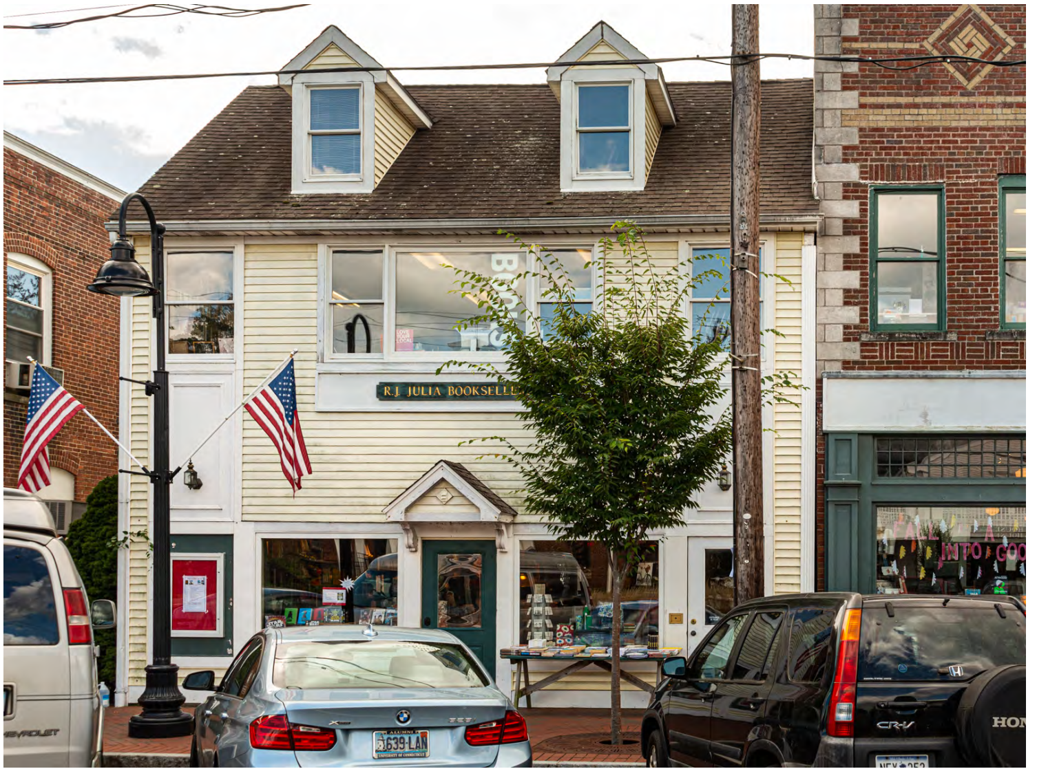
Photo 1. View south showing facade.
