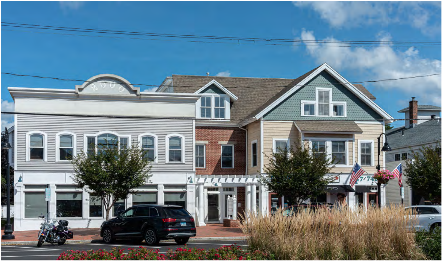
Photo 1. View north showing facade.
