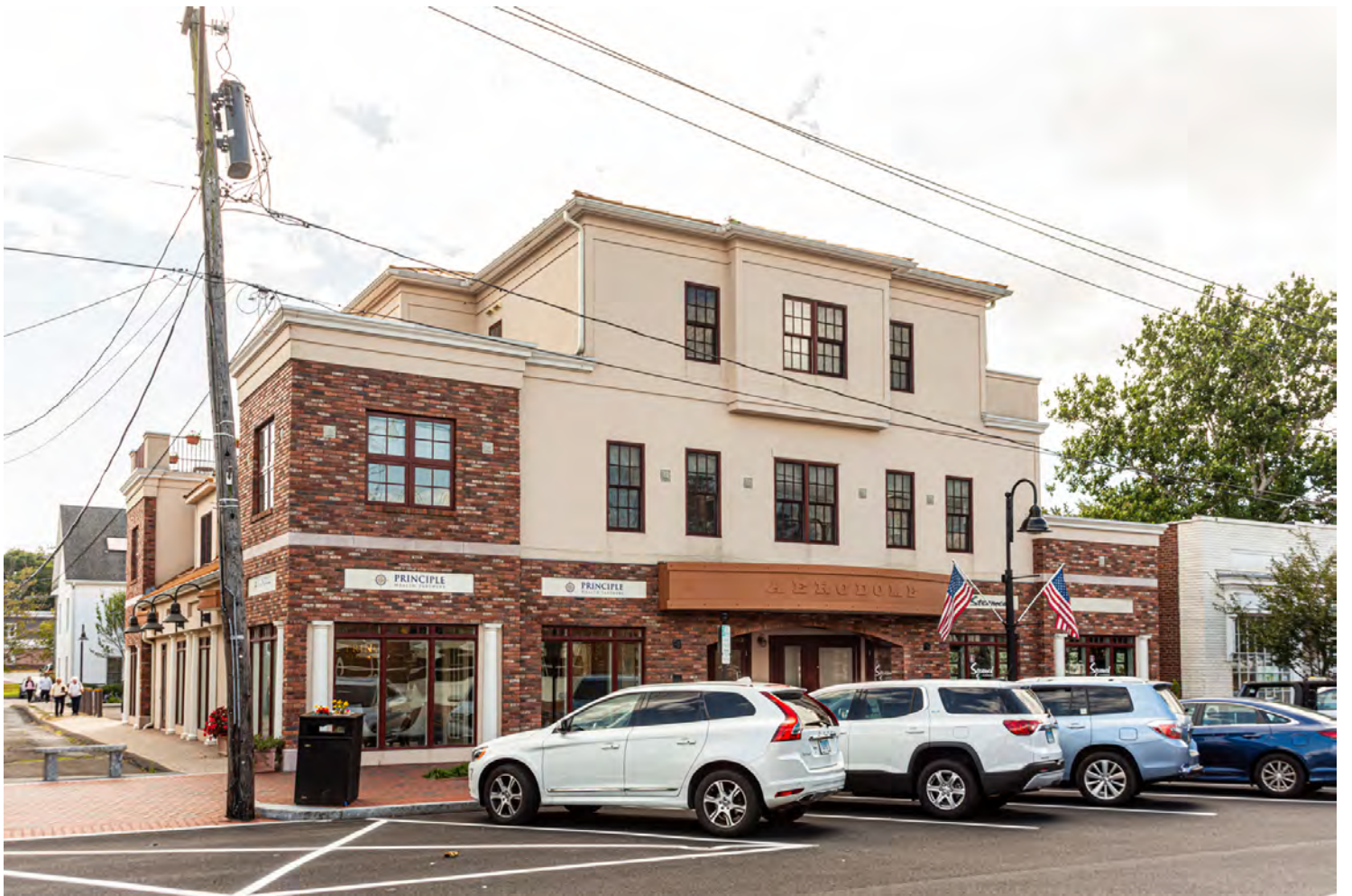
Photo 1. View southeast showing north elevation and facade.
