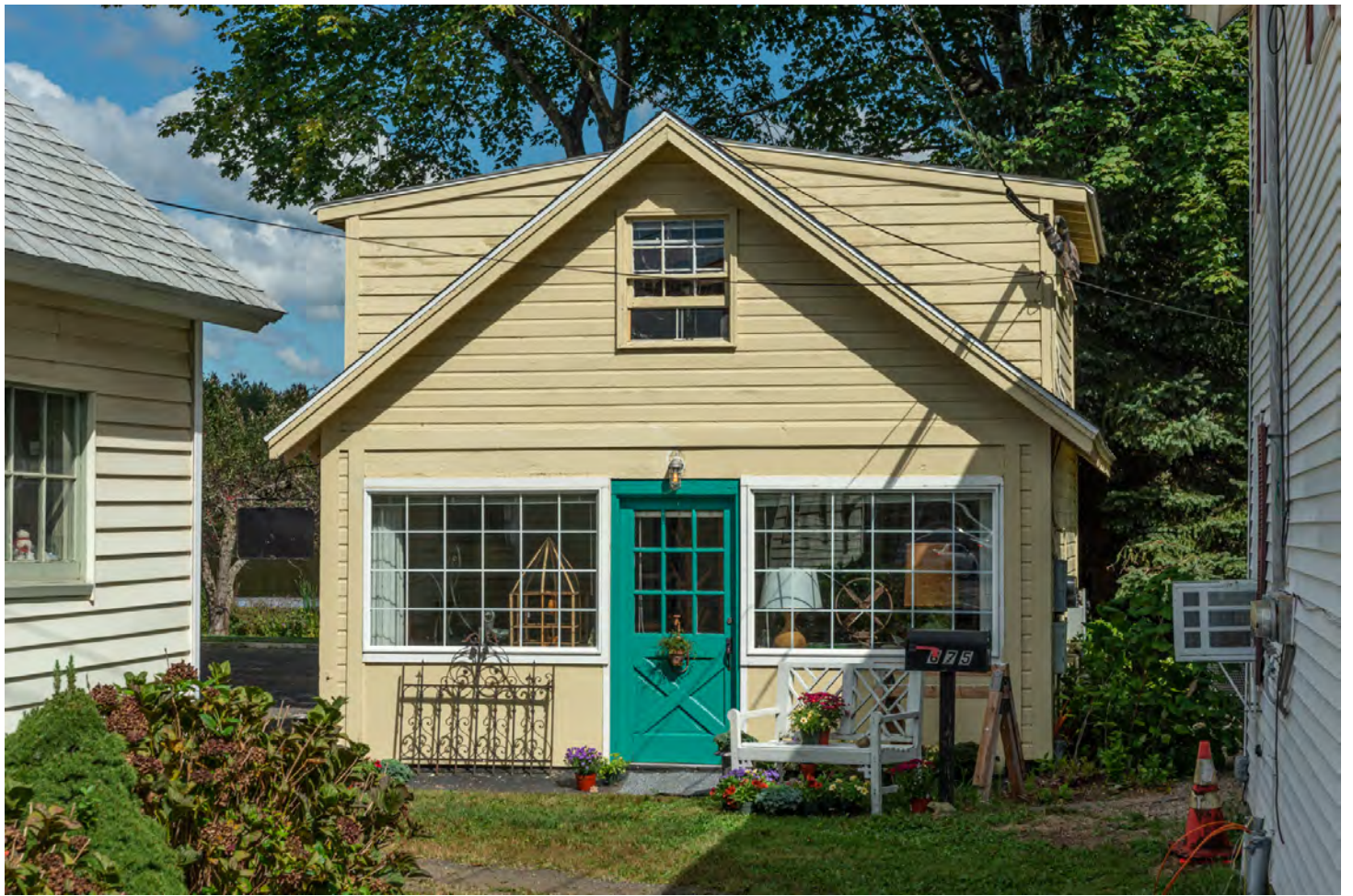
Photo 1. View north showing facade.
