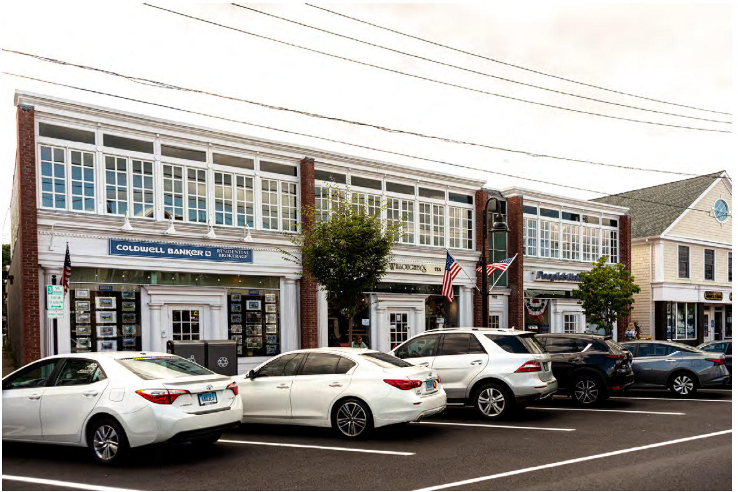
Photo 1. View southwest showing facade.
