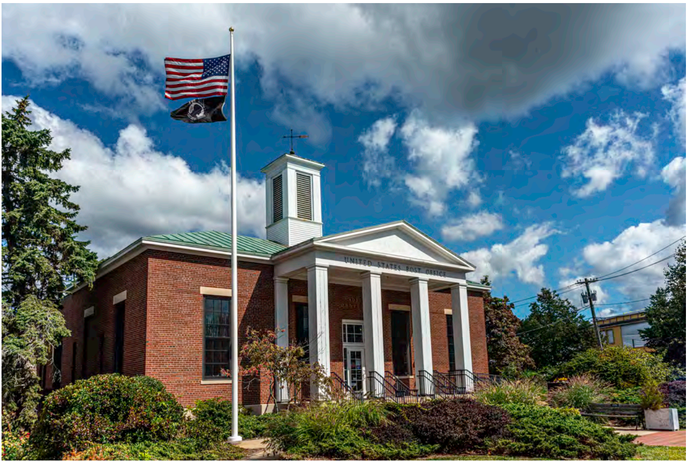
Photo 1. View northeast showing part of west elevation and facade.
