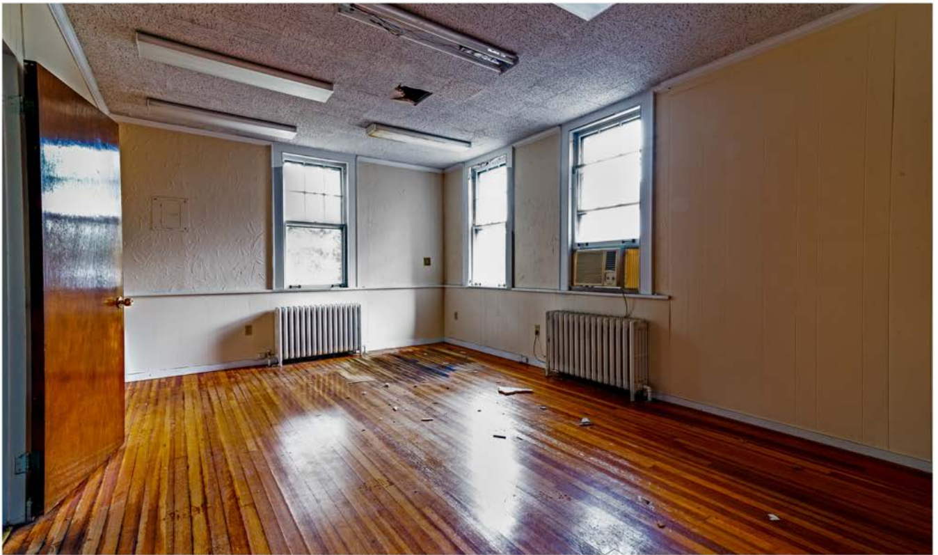
Photo 22. Interior view south east showing east end of south office on second floor.
