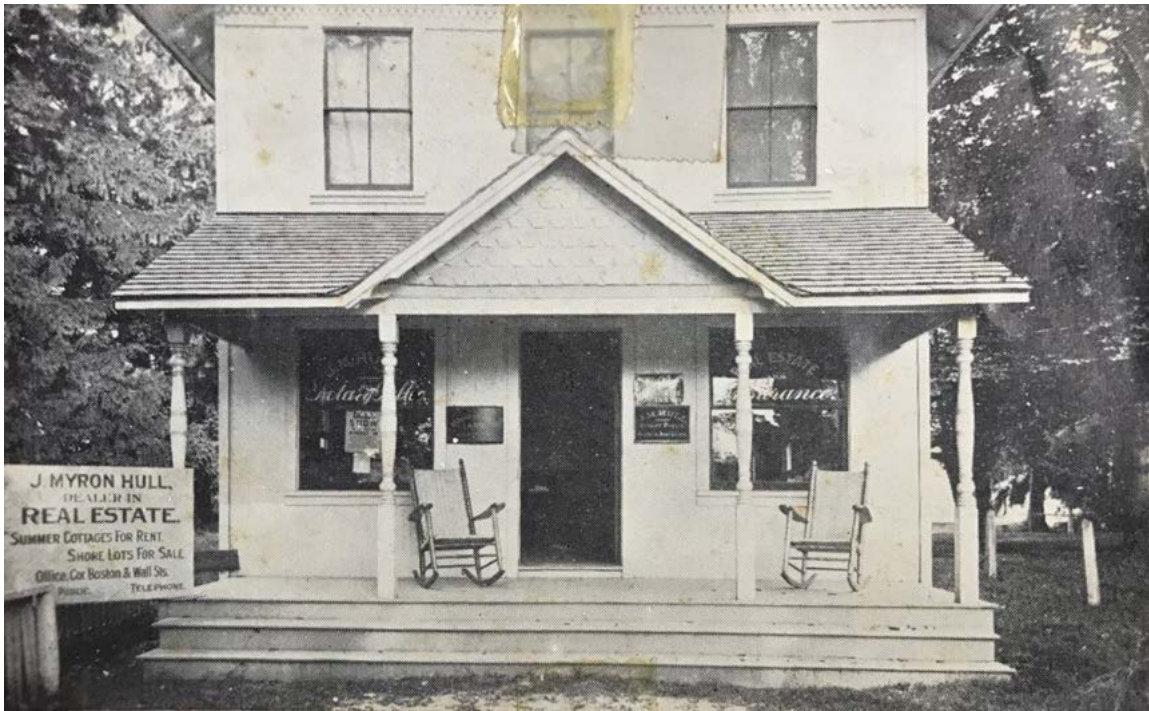
Figure 4. Façade of first hull building c.1920. (Charlotte L. Evarts Memorial Archive)
