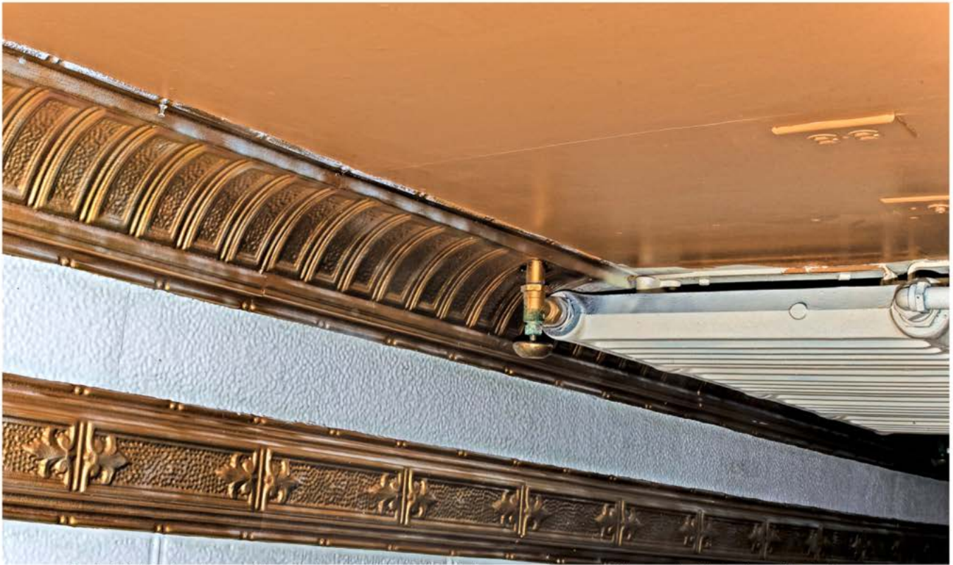
Photo 13. Interior view southeast showing stamped metal crown moldings, ceiling and radiator in north retail space.
