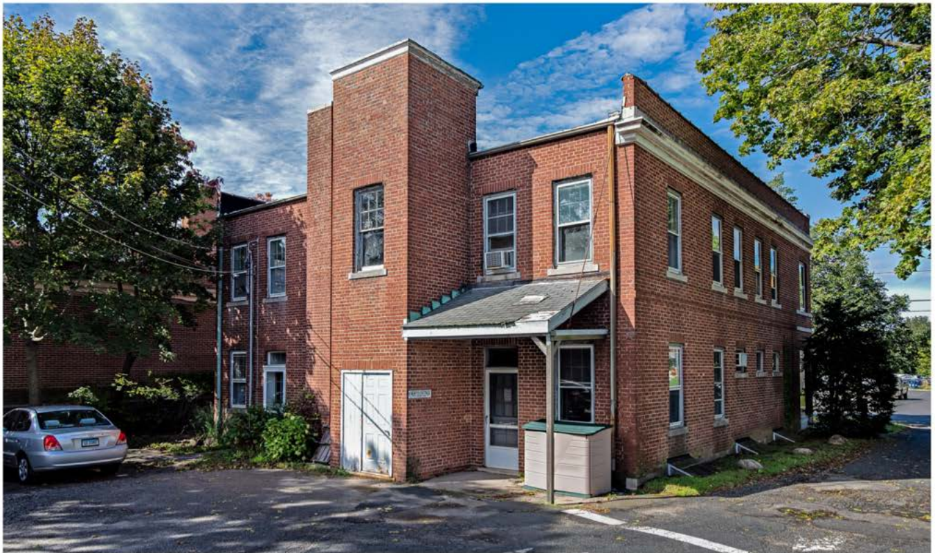
Photo 8. View southwest showing east and north elevations.
