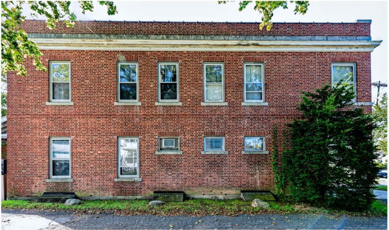
Photo 7. View south showing north elevation.
