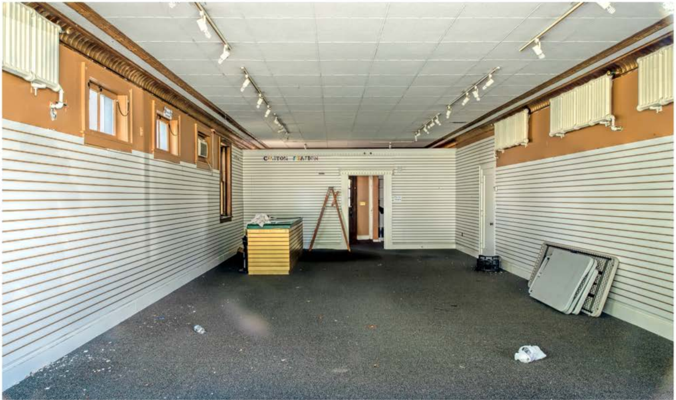
Photo 11. Interior view east showing eastern section of north retail space.
