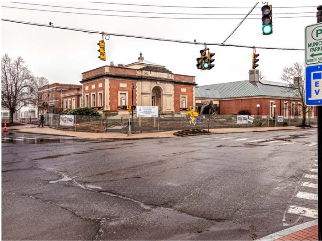
Photo 1. View north showing facade of Hull Building and E. C. Scranton Memorial Library at the intersection of Wall Street and Boston Post Road.
