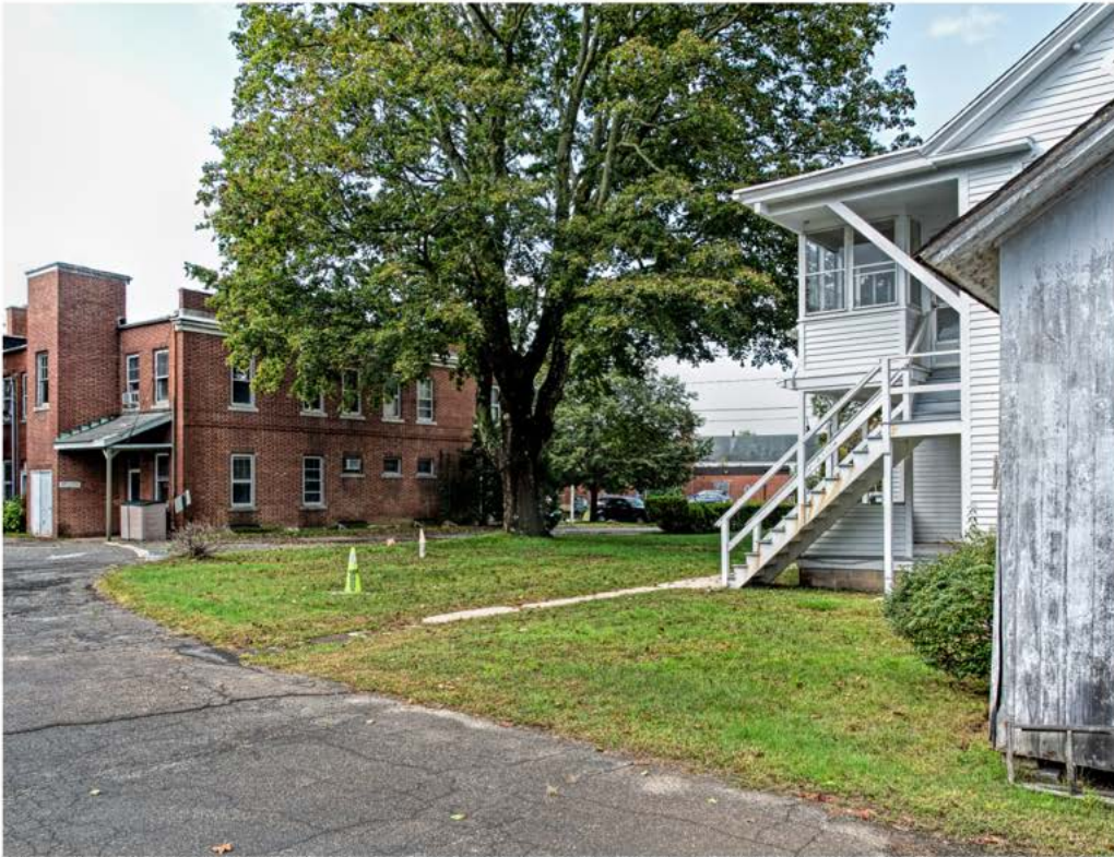
Photo 5. View southwest showing residence to the north of the Hull Building, north and east elevations
