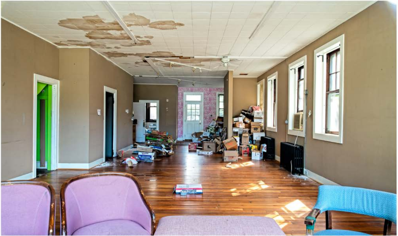
Photo 14. Interior view east showing south retail space.
