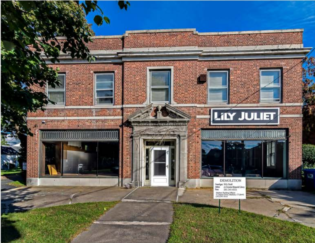
Photo 3. View east showing facade of the Hull Building, paved areas and lawn.
