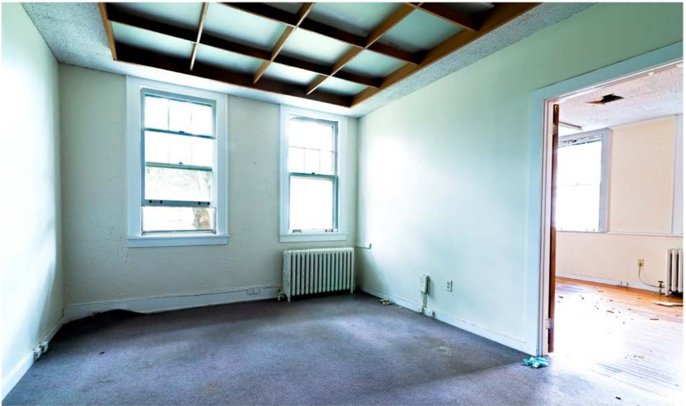
Photo 20. Interior view southeast showing east end of south office on second floor.
