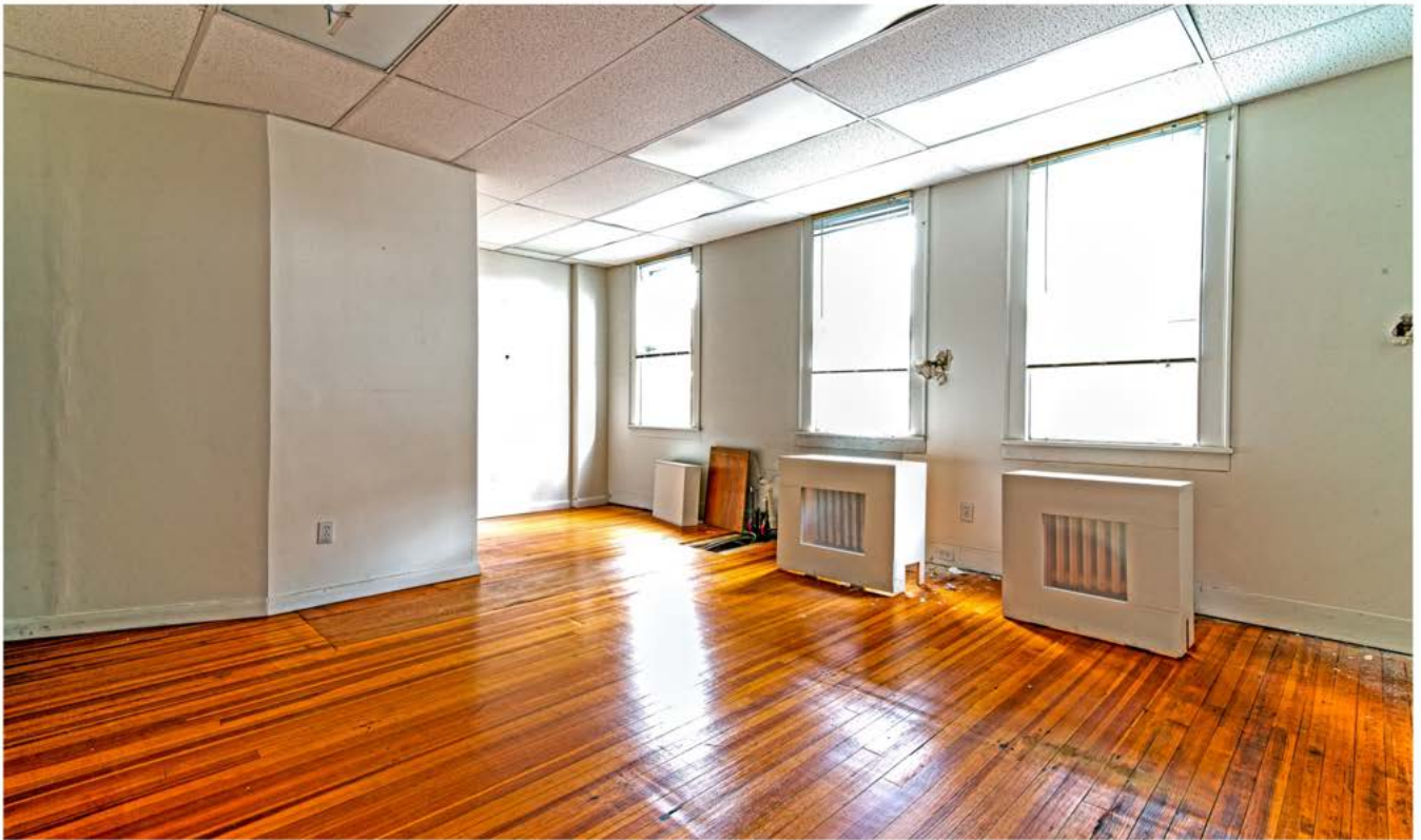
Photo 21. Interior view northeast showing center section of south office on second floor.
