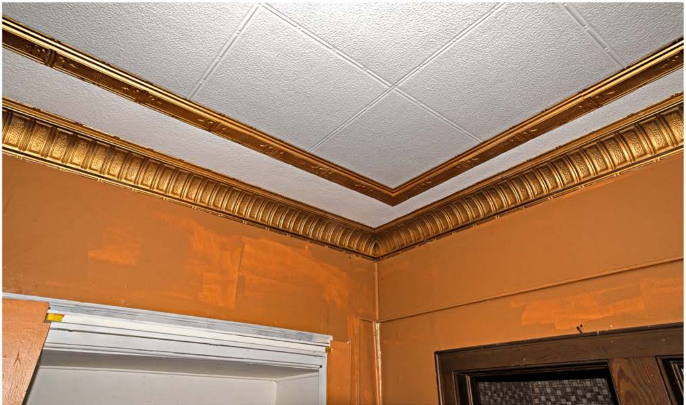
Photo 12. Interior view southeast showing crown molding on south eastern section of north retail space.
